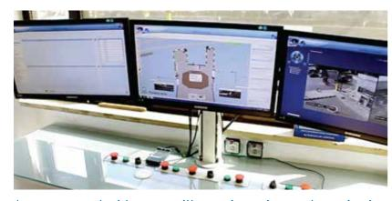
Access control, video surveillance, intrusion and monitoring Control Centers, multidisciplinary and suitable for 24x7 operation.
